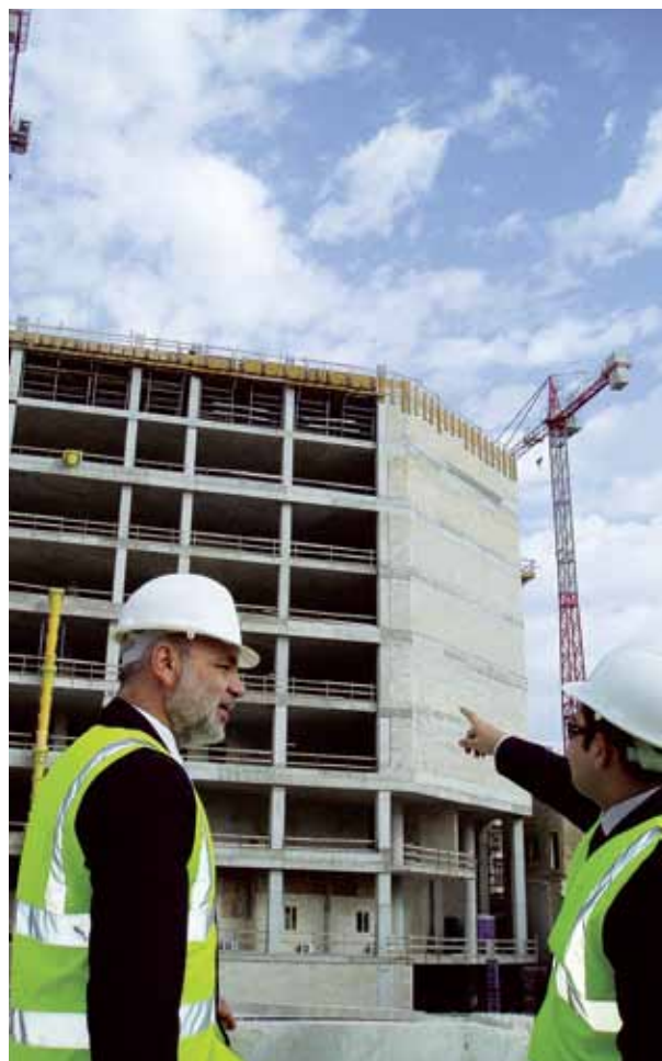
Employees monitoring progress of the new Head Office.
